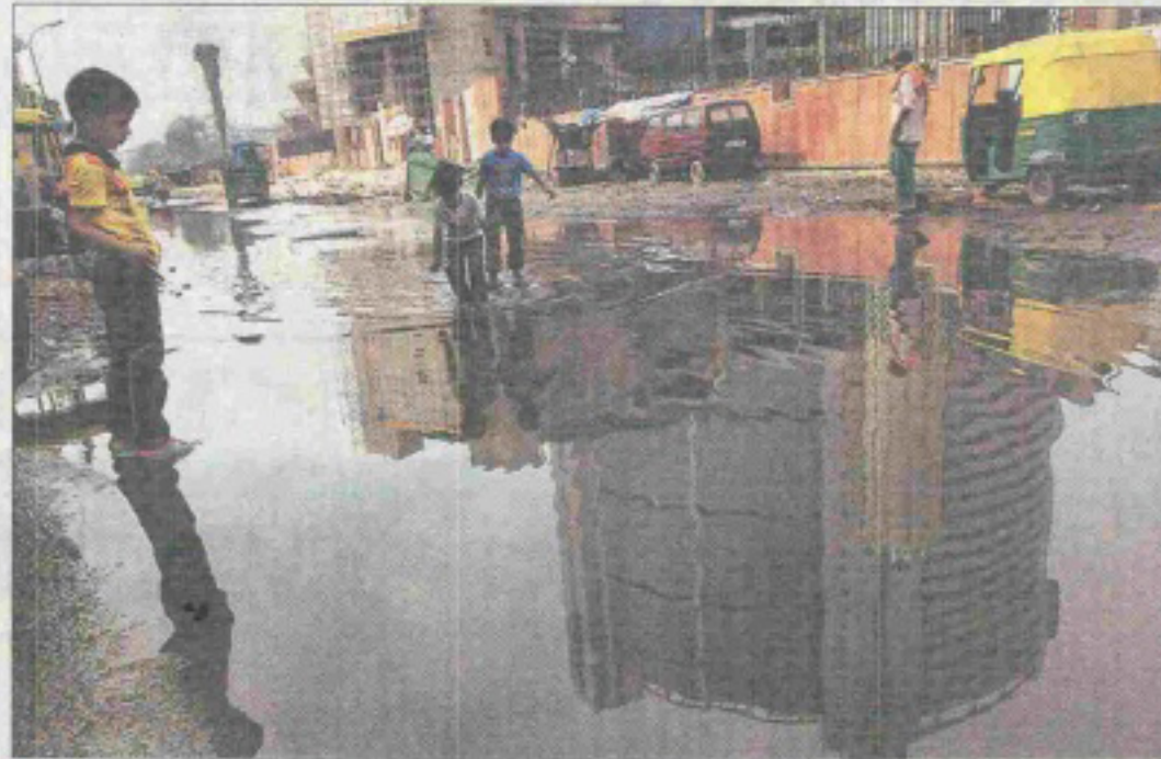
Despite the Capital facing a dengue outbreak, the authorities have yet to clean up the water collected in this stretch behind the MCD's Civic Centre. SONU MEHTA/HT PHOTO
